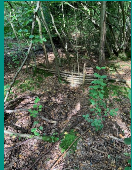
Leaky dams installed in Park Wood, October 2023 (Source: Hillingdon LLFA)
