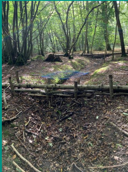
Leaky dams installed in Park Wood, October 2023 (Source: Hillingdon LLFA)
